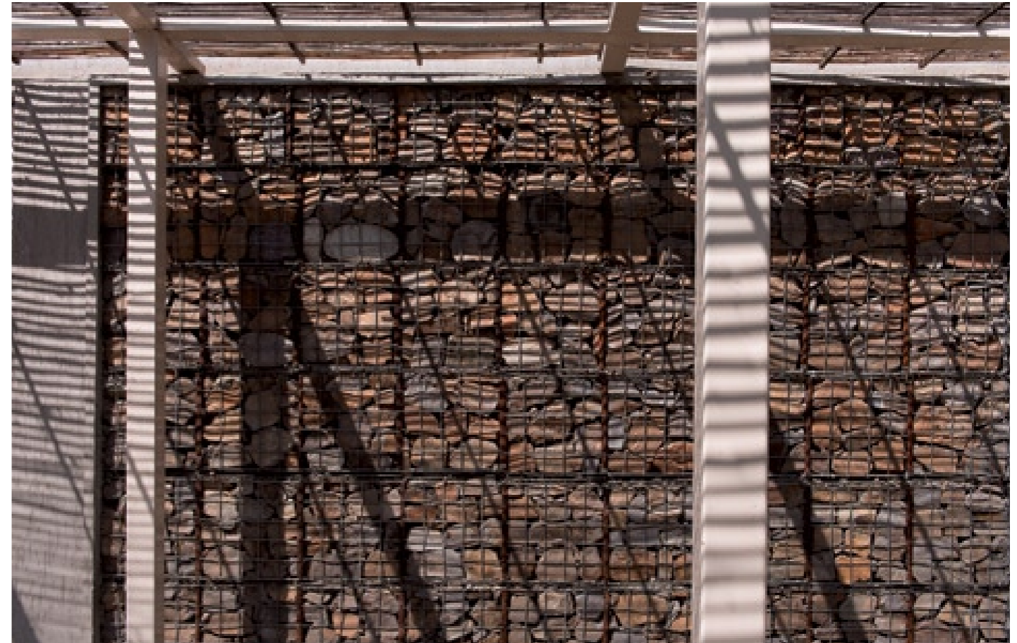
The gabions are filled with rocks from the site itself, as well as polished riverstones.
